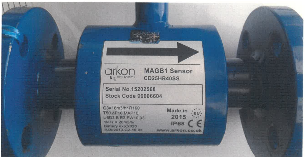
Figure 4: An example of the label and sealing:
